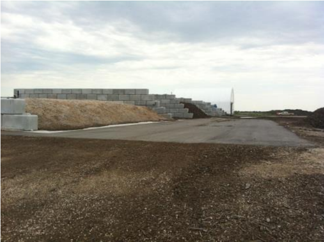
Process air to biofilter for odour treatment
